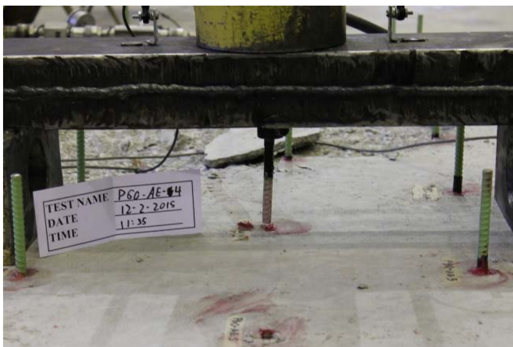
Figure B.42 Detailed view of the reinforcement at failure for P60-AE-5
