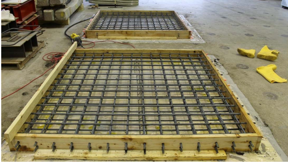
Figure 3.5 Rebar preset before the concrete placement
