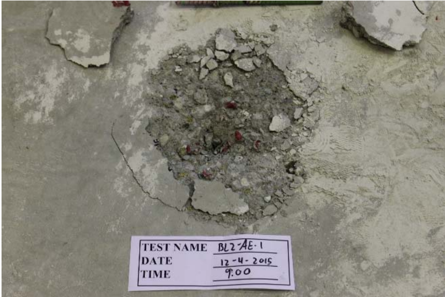
Figure 4.10 Representative failure mode for BL-AE of combined failure (concrete breakout and steel rupture)
