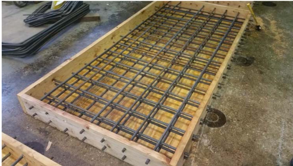
Figure 3.2 Rebar preset before the concrete placement
